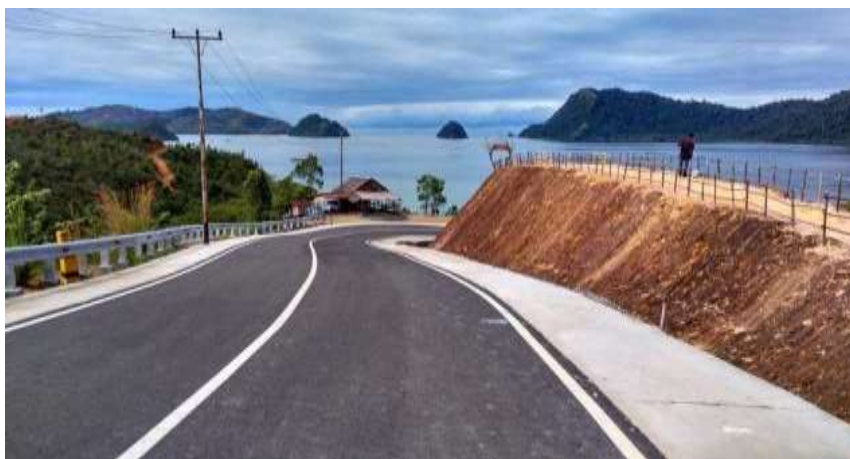
Figure 6. Road Conditions Leading to Mandeh Island Village
