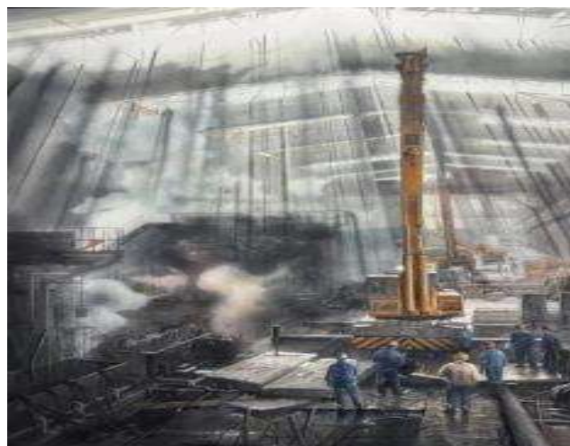
Figure 10 Kong Lingfa's work: Construction at Dawn (晨光中的建设).
